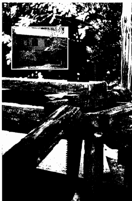
Logs from Flomaton were used for restoration purposes in Colonial Williamsburg. Here tree #281, determined to be 287 years old, is cut to be used in the Peyton Randolph home (Inset).
