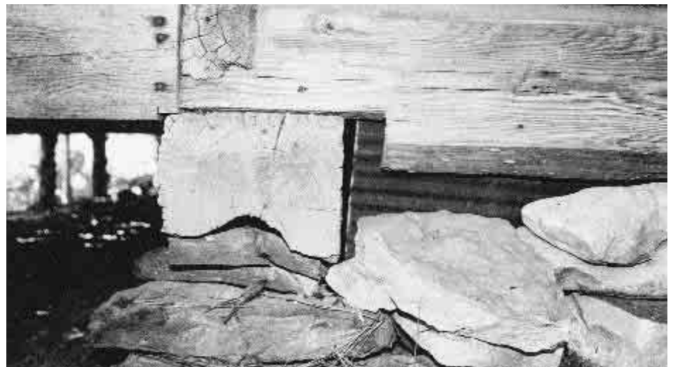
Sill logs are the large, hand-hewn logs that form the bottom of the house. They are not notched, but joined flush to create a stable foundation.
