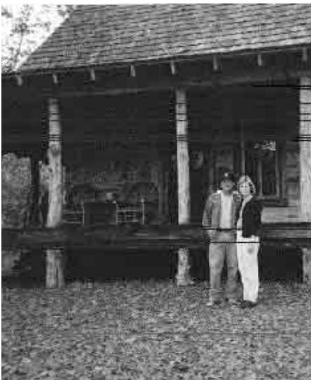
Shelby County TREASURE Forest landowners Mike and Cathy Strong have restored several log structures.
