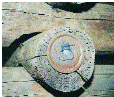
This simple numbering system was used on a corncrib relocated a few years ago.
