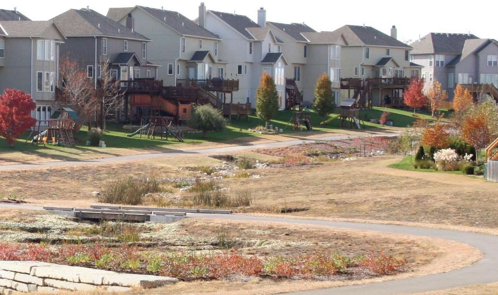
A constructed waterway and wetland in a new housing development slows delivery of stormwater and provides some initial water quality treatment as the water interacts with plants and soil. This location also contains interpretive signs along the public walkway.
